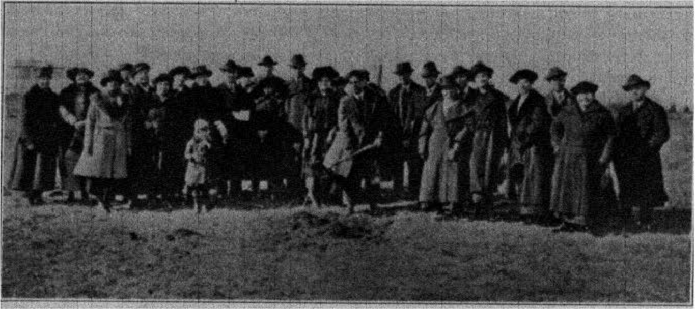
Friends assembled on Mashriqu'l-Adhkár grounds, Chicago, March 21, 1921. Dr. Zia M. Bagdádí digging first shovelful of earth.
